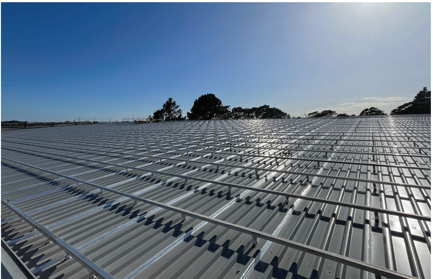
RL LinerDeck with Post & Rails during installation
