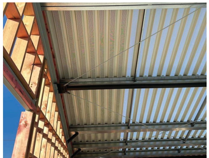
RL Perforated LinerDeck during installation
