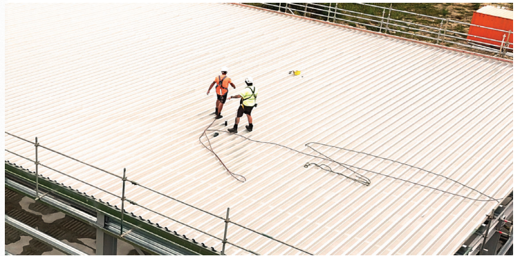
RL LinerDeck during installation
